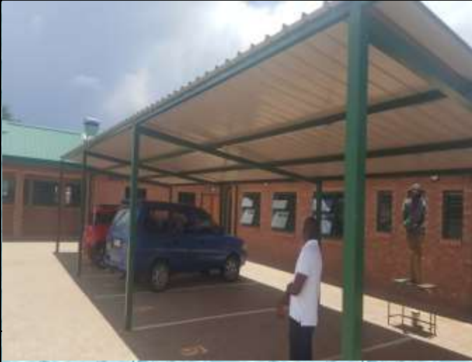
MANKHOLE SECONDARY SCHOOL
